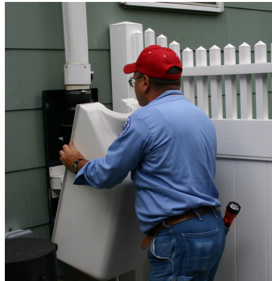
Figure 6-1 Inspection of SSD fan and weatherproof
