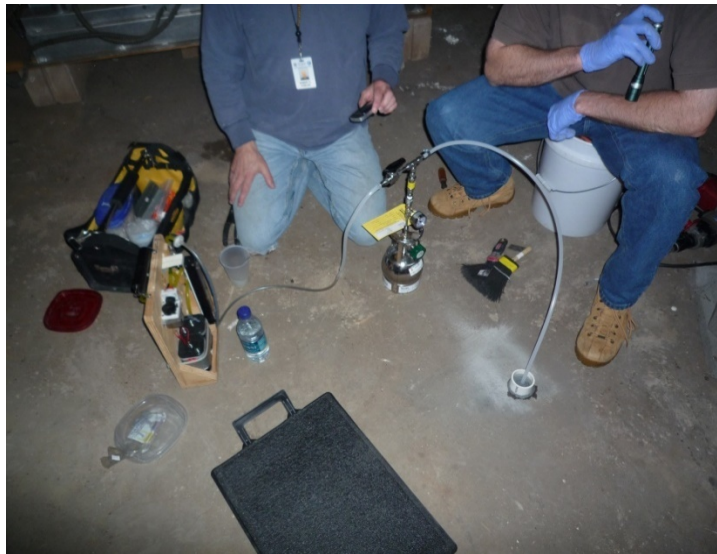
Figure H-3 SSP evacuation with pump, in-line “T” fitting and water dam leak check (NJDEP)
