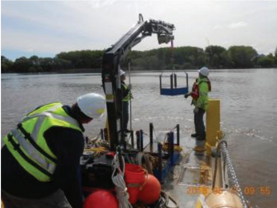
FIGURE 12 Cap thickness verification using catch pans.
