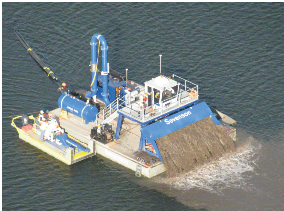
FIGURE 7 Hydraulic cap placement using Sevenson's spreader barge. Photo courtesy of Sevenson Environmental.
