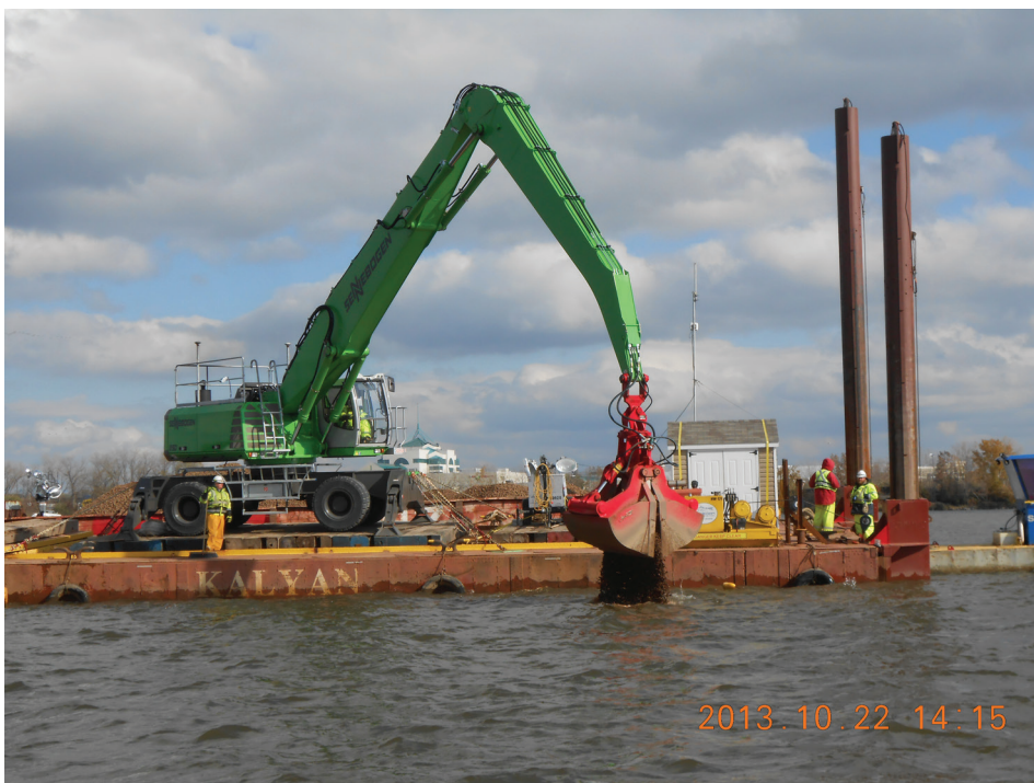
FIGURE 6 Mechanical cap placement.
