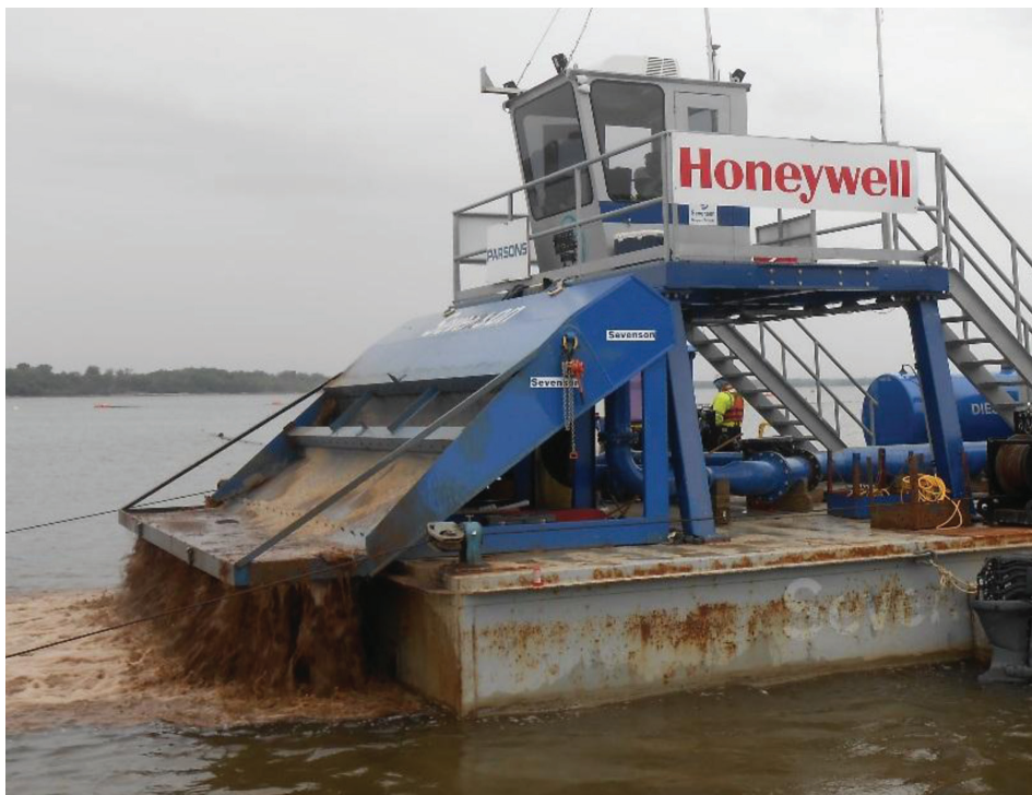
FIGURE 10 Metal grate modification on spreader barge.
