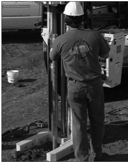
Figure 4.25. The sampler should be parallel to the probe derrick for driving.
