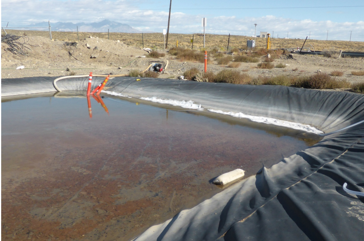
Figure 8. AFFF contaminated lagoon water.
